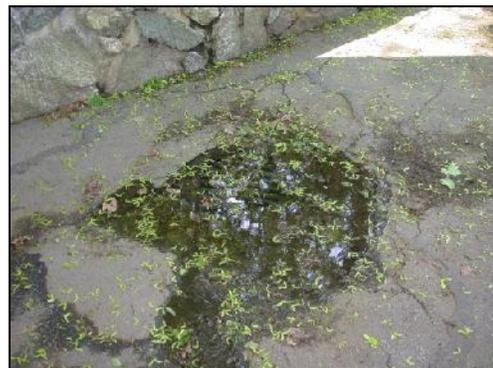
*But a hose test proved the drain was non-functional*
