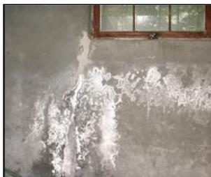
*Efflorescence on a concrete garage wall*
