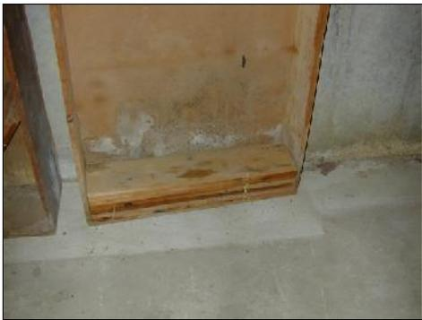
*Mold on a shelf that has been stored up next to cold concrete*
