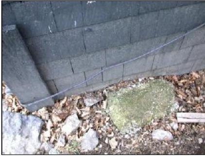
Wood/soil contact at an exterior wall
