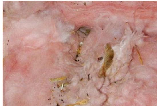
*Mouse droppings and burrows in exposed fiberglass insulation*
