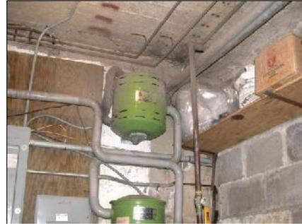
**Dust from leaky central vacuum canister**
