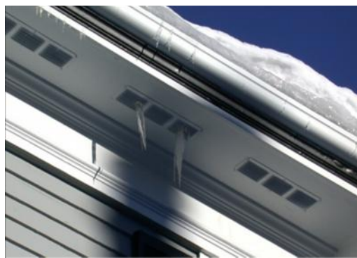
Ice dam water in soffit May Indoor Air Investigations LLC
