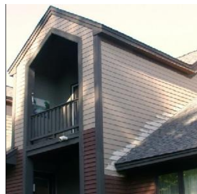
Cement-board siding, peeling shingles
