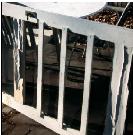
Paint peeling from a screen door May Indoor Air Investigations LLC
