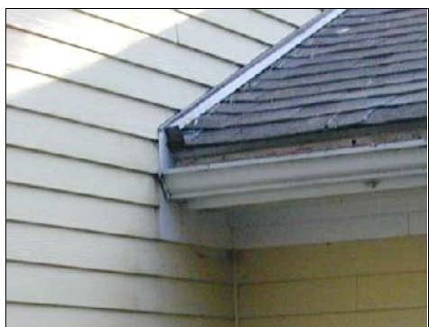
Cement-board kick-out flashing May Indoor Air Investigations LLC
