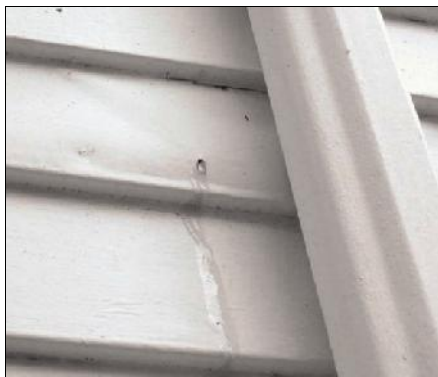
Water leaking from a paint blister May Indoor Air Investigations LLC
