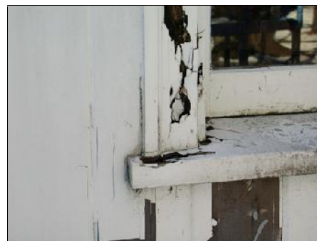
Peeling paint and decay resulting from incorrectly sloped window-cap flashing May Indoor Air Investigations LLC
