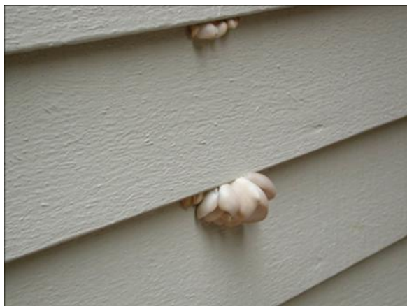
Mushroom growing out of siding due to moisture behind the cladding
