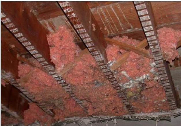
*Rodent burrows in fiberglass insulation*
