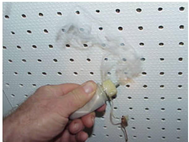
Sometimes there are gaps between the wall and plumbing access panel. Or even worse - the panel is made from peg board to enhance transfer between units..
