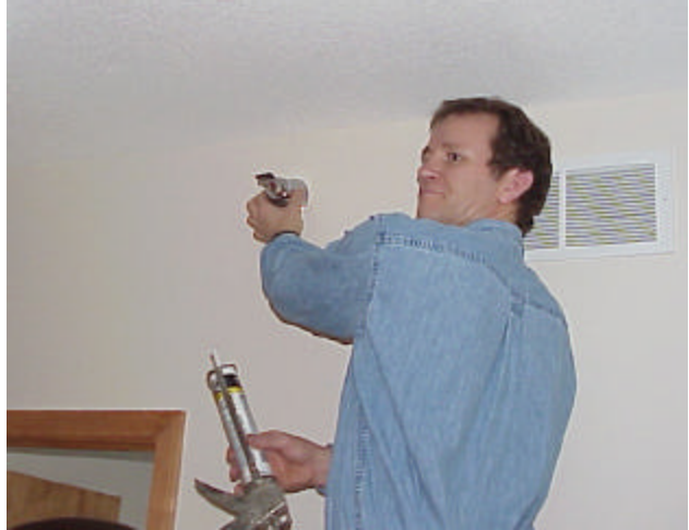
Caulk used to seal around pipe
