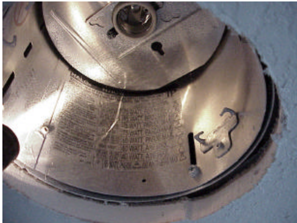
Large leak in and around recessed light fixture (4 Story building)
