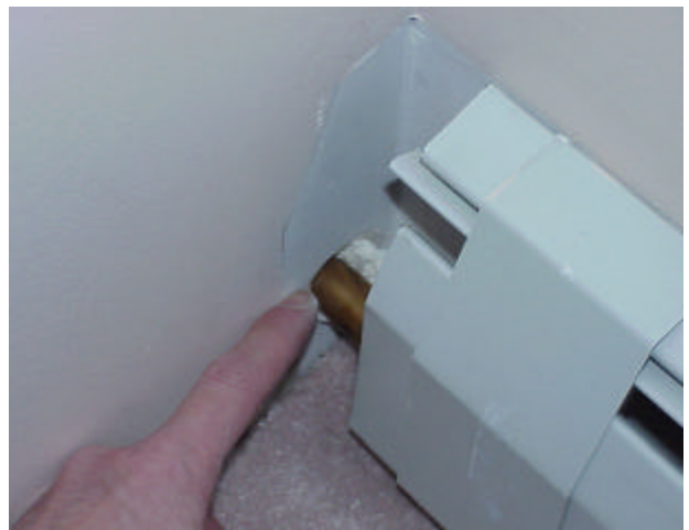
Foam used to seal gap around pipe
