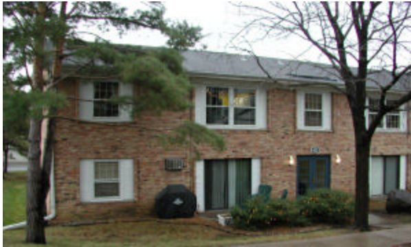
Figure 13. Building 8-Plex exterior photo and first floor plan
