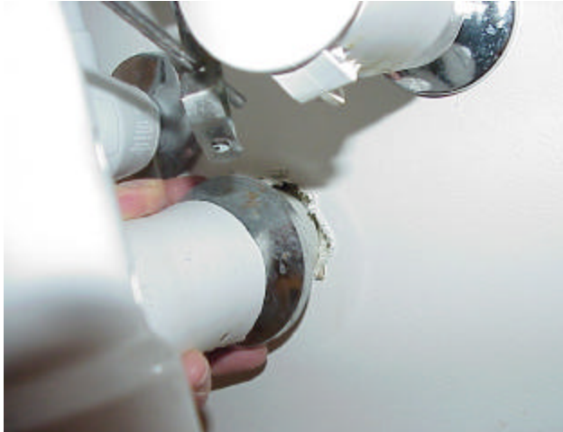
Moderate-sized wall gaps around bathroom/kitchen plumbing (138 Unit building)
