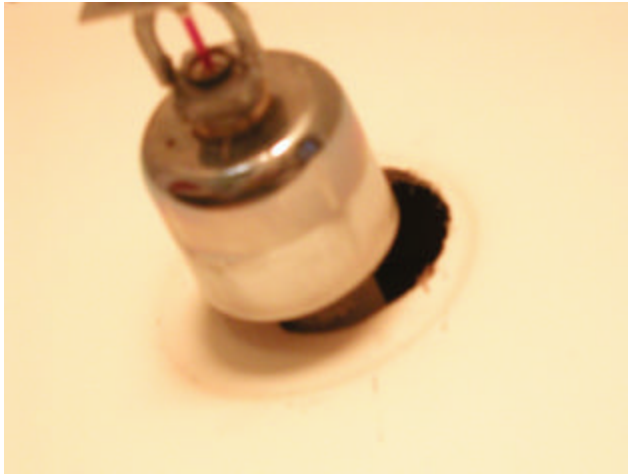
Open gap around sprinkler pipe (4 Story building)
