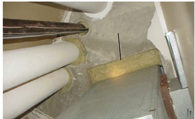
Mineral wool applied into large gaps
