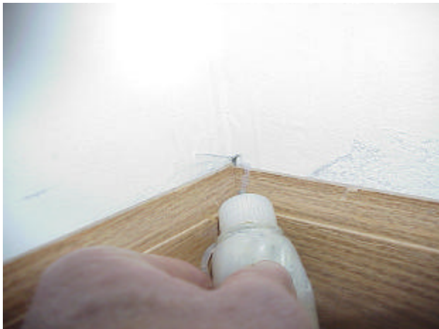
Smoke movement into gap behind baseboard (138 Unit building)
