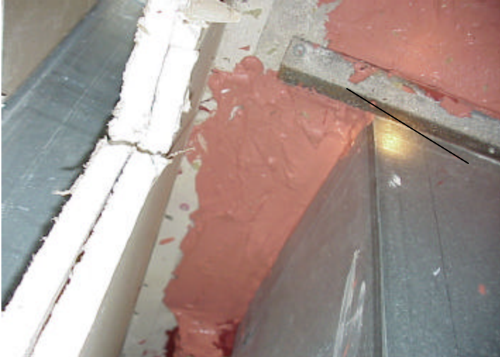
Seal with listed fire barrier
