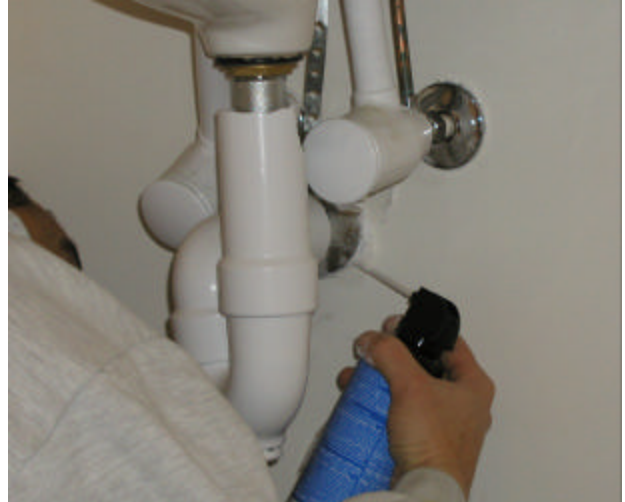
Foam used to seal around the gaps
