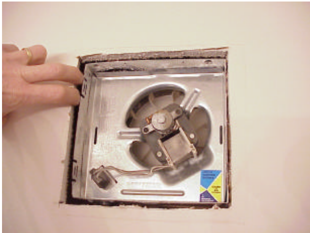
Significant wall gaps around bathroom exhaust fan housing (4 Story building)
