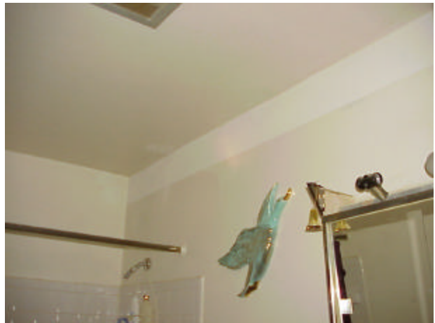
Wall patched and ready for final coat of paint
