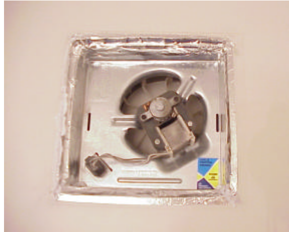
Gaps sealed with caulk and metal tape
