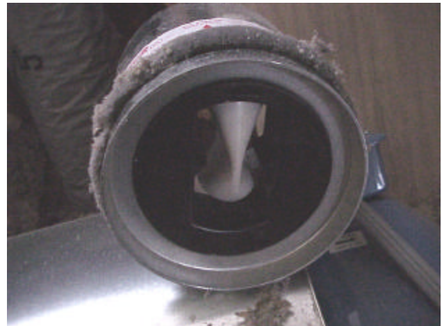
Figure 22. Constant air regulator installed at manifold inlets
