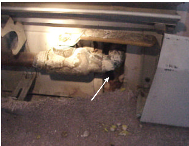
Large gap in wall between units for hydronic heating pipe (11 Story building)
