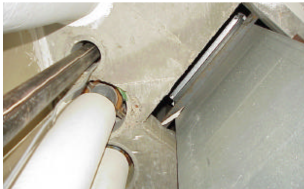
Looking down at large gaps around metal duct and pipes in a mechanical chase (11 Story building)
