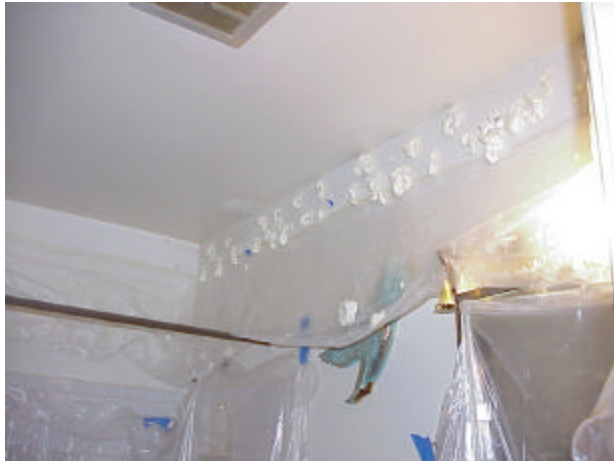
Foam injected at top of open plumbing cavity to create continuous plug to stop air movement up cavity (12-Plex building)
