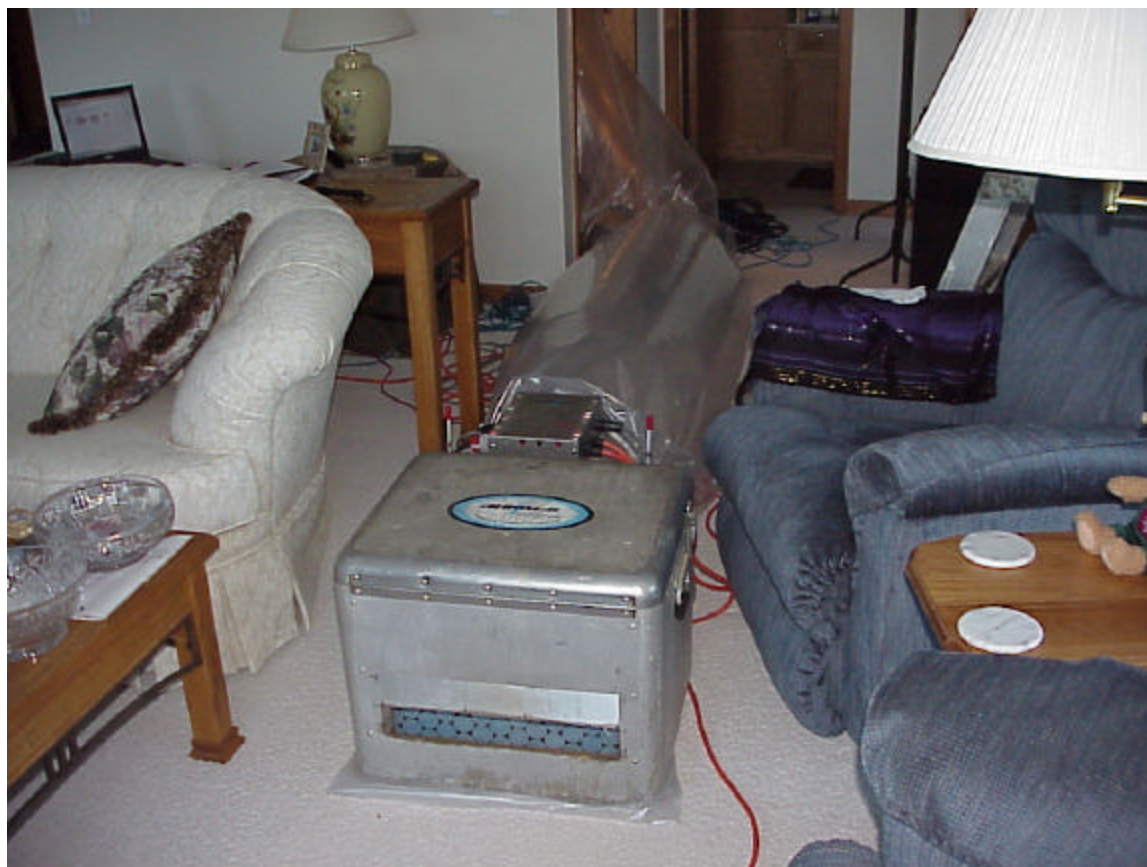
Figure 20. Duct sealing aerosol injection system
