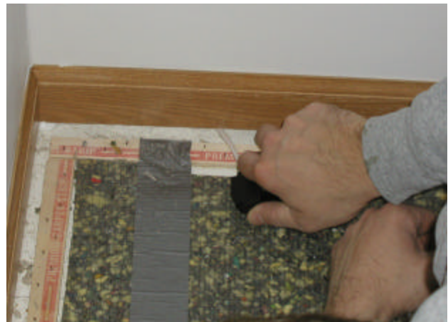
Foam treatment for large gap. Smaller gaps treated with clear acrylic caulk.
