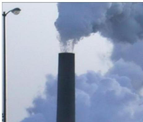
*Vapor condensing to liquid to create cloud droplets. Note clear zone of vapor at stack top.*
