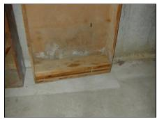
Mold on set of shelves; note efflorescence at bottom of foundation wall May Indoor Air Investigations LLC
