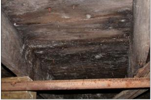
Mold growth on joists and subfloor in unfinished basement due to elevated relative humidity
