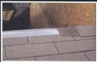
As a worst-case comparison, the attic ridge was sealed with duct tape and ridge cap shingles. The attic temperature rose 65.8°F
